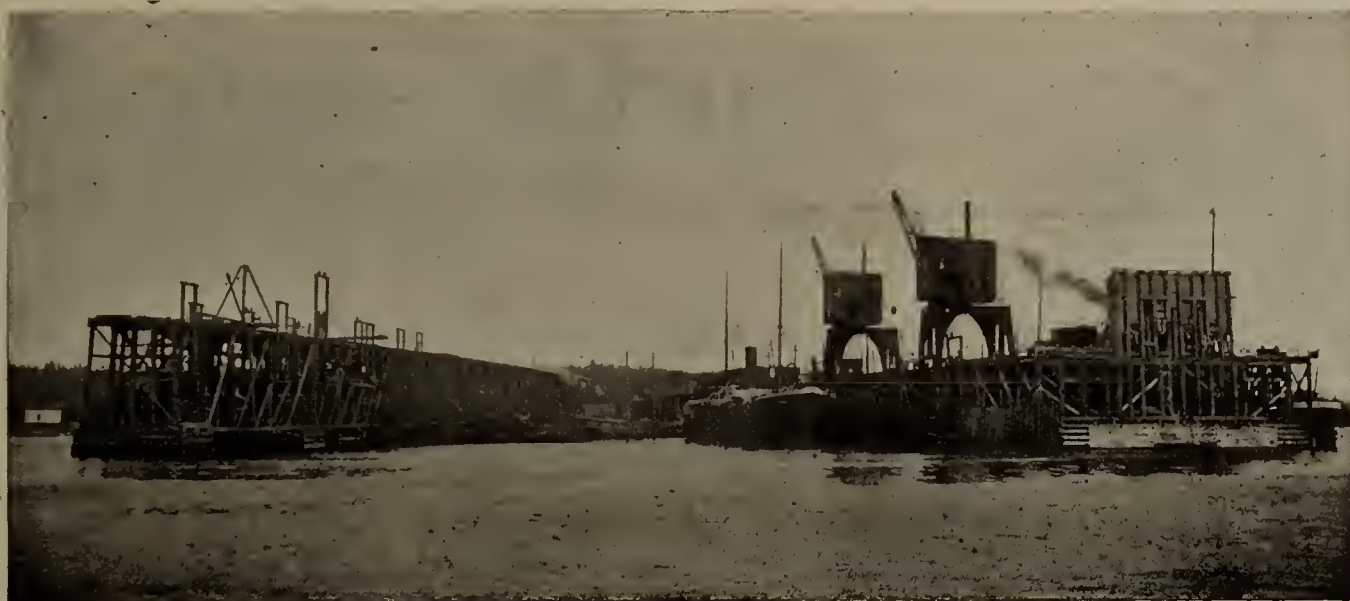
International Shipping Piers of the Dominion Coal Co., Limited, at Sydney, C.B.
